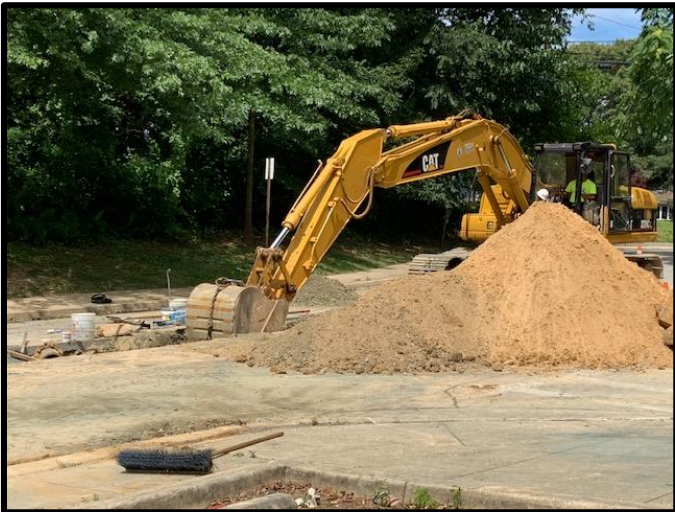
Water Line Installation
